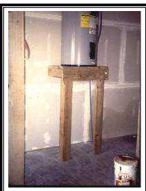
This wet floodproofed garage has bare concrete, unfinished drywall (for fire protection), and an elevated water heater.
